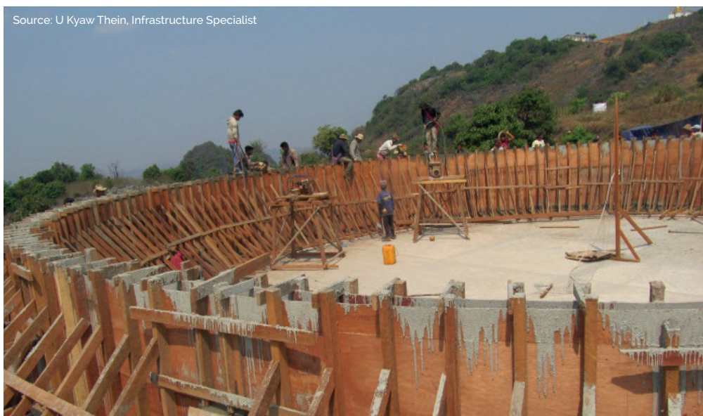
80,000 gallon capacity collector tank under construction, Pinlaung Township
